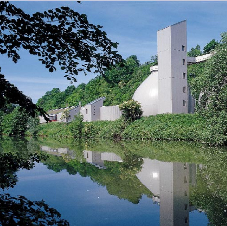
Tübingen sewage plant
