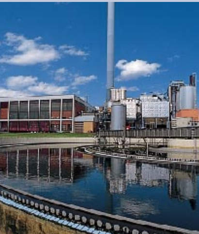
Stuttgart Mühlhausen main sewage plant
